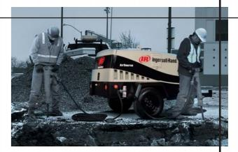
**AirSource is ideal for two-tool applications.** The AirSource is designed to provide sufficient power to two tools simultaneously. With an output of 160 cfm and a pressure range of 80 - 125 psig, the AirSource is an exceptional value that allows you to meet even the toughest jobsite demands.
