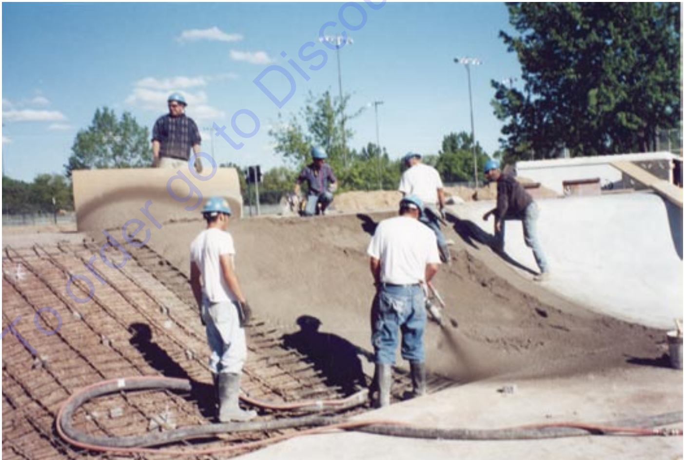
Shotcreting (wet gunning) with a stiff, low-slump shotcrete mix is all in a day's work for the Mayco C30HDN.
