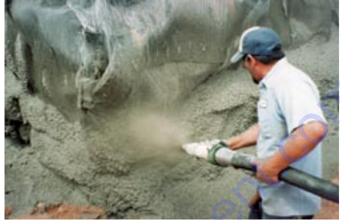
The C-30HD series is ideal for shotcrete applications of stiff, low slump mixes — swimming pools, ditch linings, soil stabilization, walls and more.
