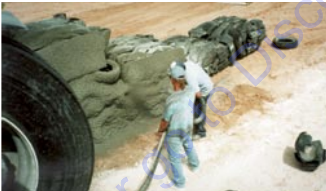
Shotcreting (wet gunning) with a stiff, low slump mix, is just one of the many uses for the LS-60 concrete pump.
