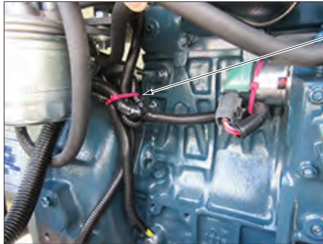
Figure 28 - Bundle and Cable-Tie Harness Wires
