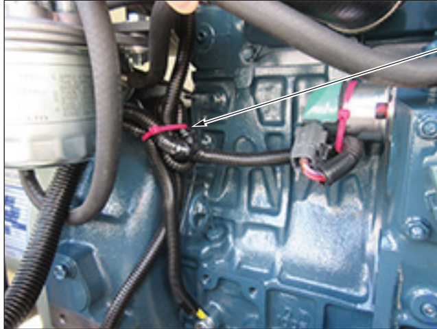
Figure 28 - Bundle and Cable-Tie Harness Wires
