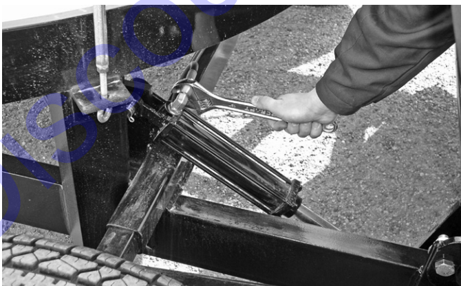
Figure B22 Loosening Hydraulic Hose Fitting to Bleed Air From System
