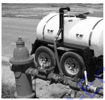
Figure B3 Filling Tank Through Anti-Siphon Fill
