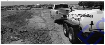
Figure B12 Side Watering Nozzle
