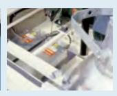
Plug-in ballasts installed in galvanized steel boxes. Can be replaced without disconnecting wiring terminals.
