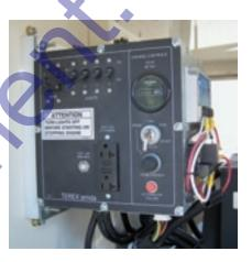
Control box shown with optional Roda Deaco electronic air shutdown system (model AL5000).
