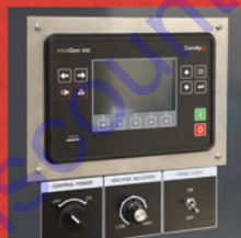
Parallelling Control Panel
