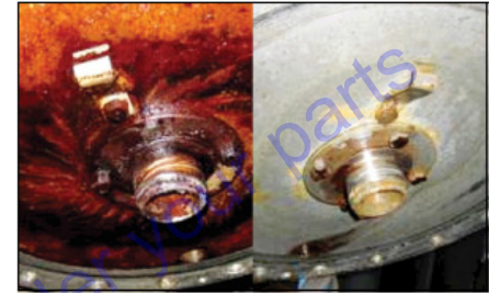
Vessel cover contaminated
