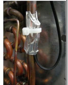
Thermistor attached to the refrigerant line.
