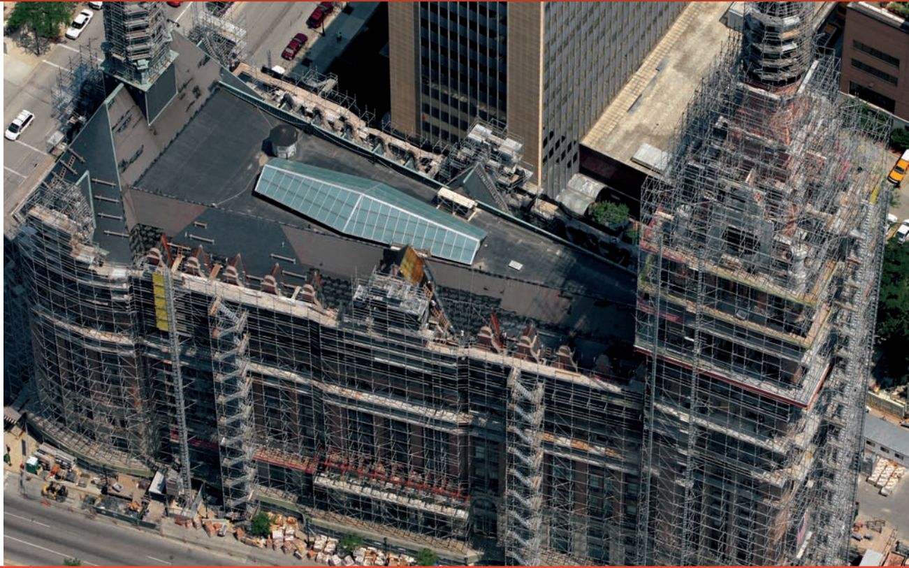
Photo courtesy of Safway, Waukesha, WI
