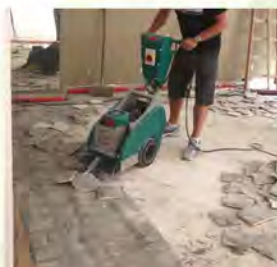
Removing ceramic tile
