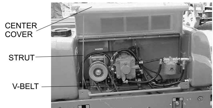
Figure 7. Checking V-Belt Tension
