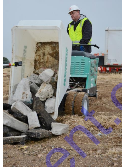
Debris removal with the WBH16AWD
