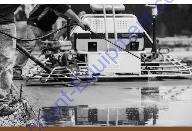
SlabArmor™ Closer is a spray-on, leave-on condensifier that dustproofs and hardens in a single application with minimal clean-up.
