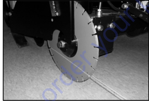
Figure 6: String Line against Blade
