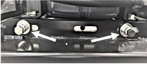
Engine Rail Bolts
