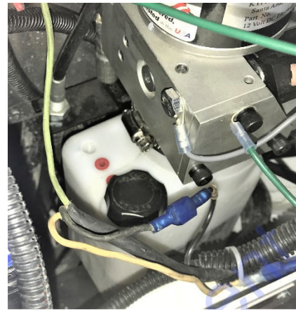
Electro/Hydraulic Pump Reservoir Cap
