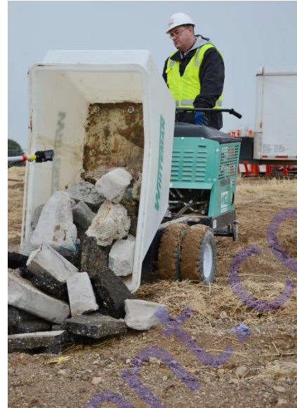
Debris removal with the WBH16AWD
