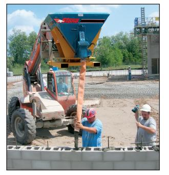
The Groutzilla™ Placement System has been Right Built for productivity and efficiency in filling block, walls and forms. It easily handles most masonry mortar and grout slumps. The mason can effortlessly swivel the hopper and move the discharge hose along the wall, filling as he/she goes; covering a substantial length of the wall before the unit needs to be repositioned.
