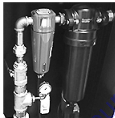
Figure 4-2. Coalescing Filter and DPI
