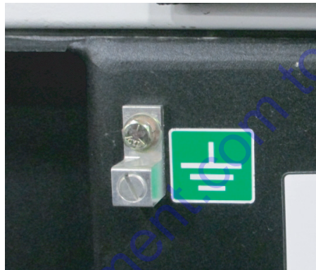
Figure 16 - Frame Ground Connection
