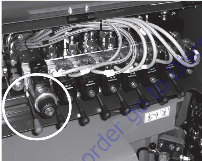
Figure 3-2. See “Ground Control Station - With Enable Lever” on page 4.
